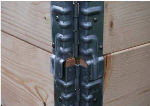
Durable hinges lock the collars firmly in place
